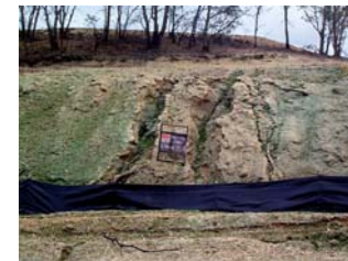
Avoid clearing vegetation or use erosion prevention and sediment control measures on steep slopes and riparian areas.
