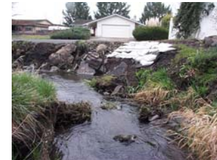
Protect riparian corridors and vegetation on stream banks to prevent erosion.
